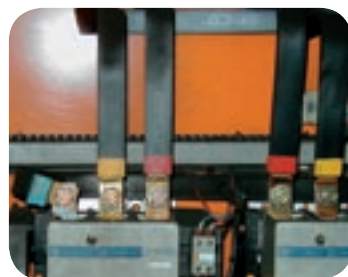
The TMTI 300 is used to inspect cable connections. The temperature of one of the cable connections is significantly higher than the others. This could indicate potential problems and should be further investigated.
